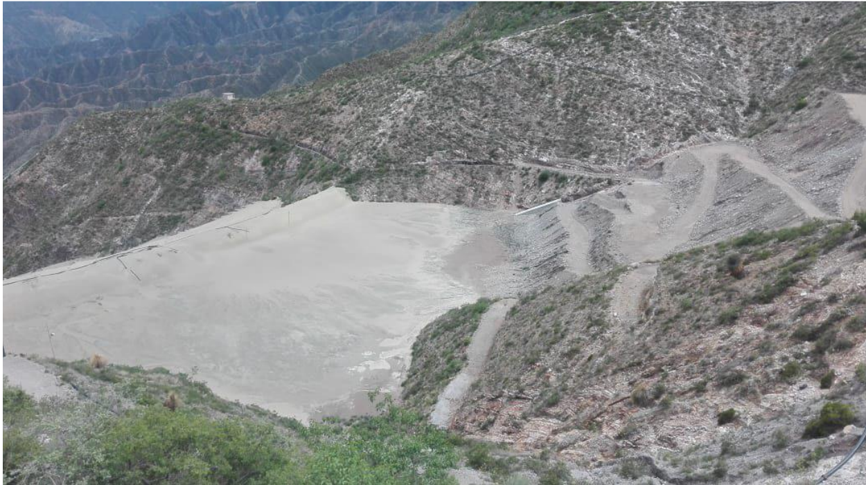
Figure 18-3 View of TSF5A (Looking Southwest - June 2021) (Britton et al., 2022)
